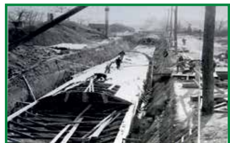
Construction of the Susquehanna Spillway tunnel to the Susquehanna River (circa 1907).
